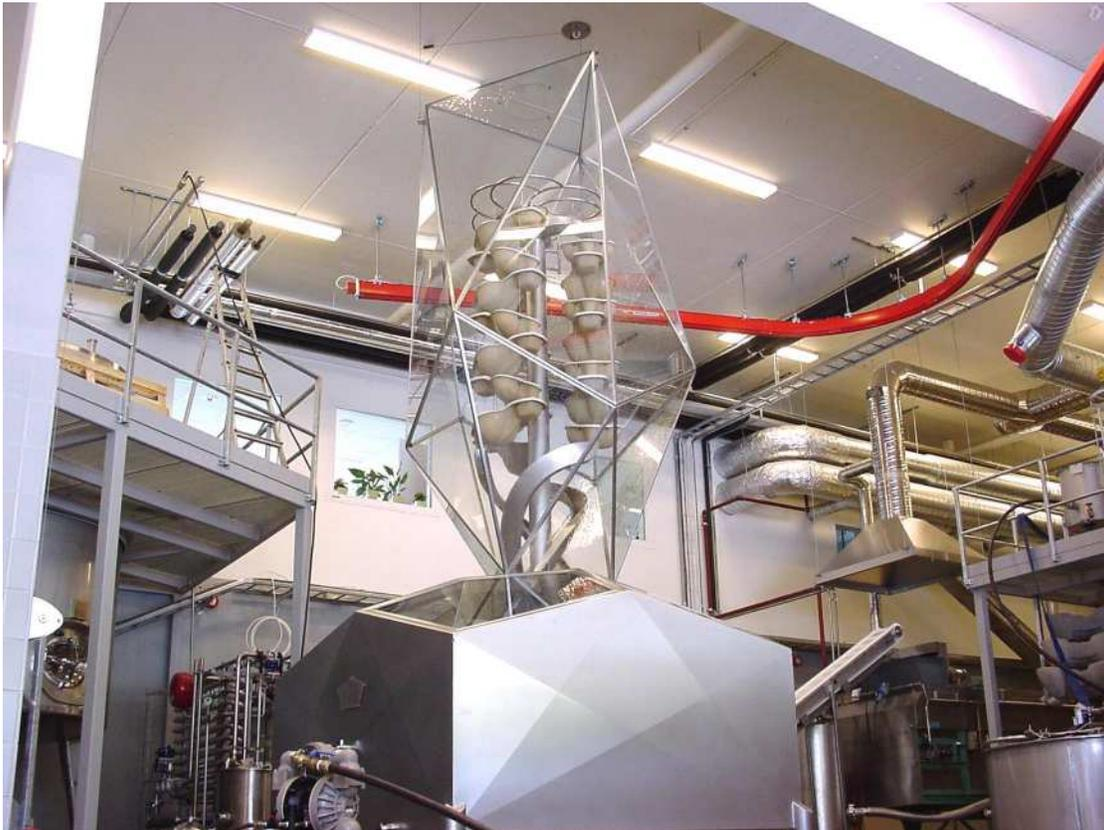
At Giubiasco in Switzerland, drinking water is gathered from springs high in the mountains for the town supply. The energy generated through falling through pipes down to the valley is extracted with a turbine and generator before it enters the municipal system. Through this process, however the water appears to become more aggressive and was attacking
